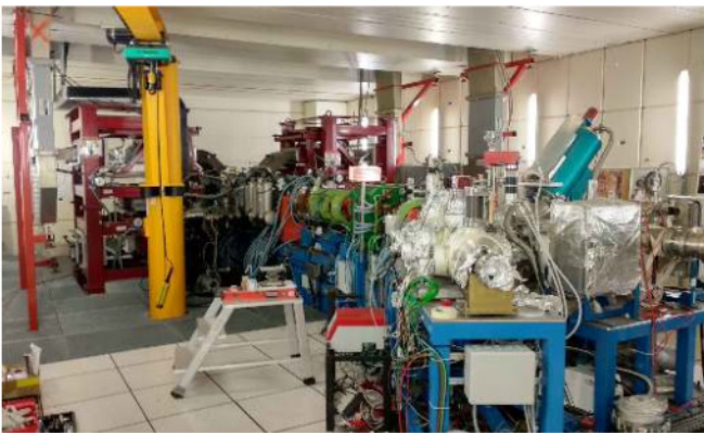
Fig. 7. Picture of the IPHI installation. The IPM test bench is also visible in the foreground.
